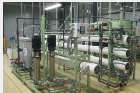
Filtration device using reverse osmosis membranes
